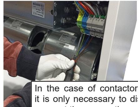
In the case of contactors, it is only necessary to disconnect the connection cables inside the curtain
