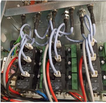
Resistance connection type for models M and ECM in all its lengths and Models G-ECG in lengths 1000 - 1500
