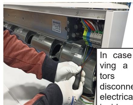
In case of having a contactors battery, disconnect the electrical wires inside the air curtain.
