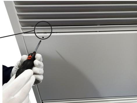
3. Raise the grate of the service door to be able to open the panel. Open the panel, being careful not to drop the grate of the service door. Once the service panel grille is closed with the service door open, open the service door fully with both hands
