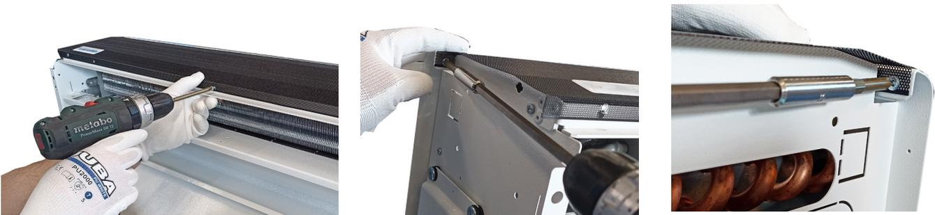
4. Unscrew the screws that hold the water coil.
